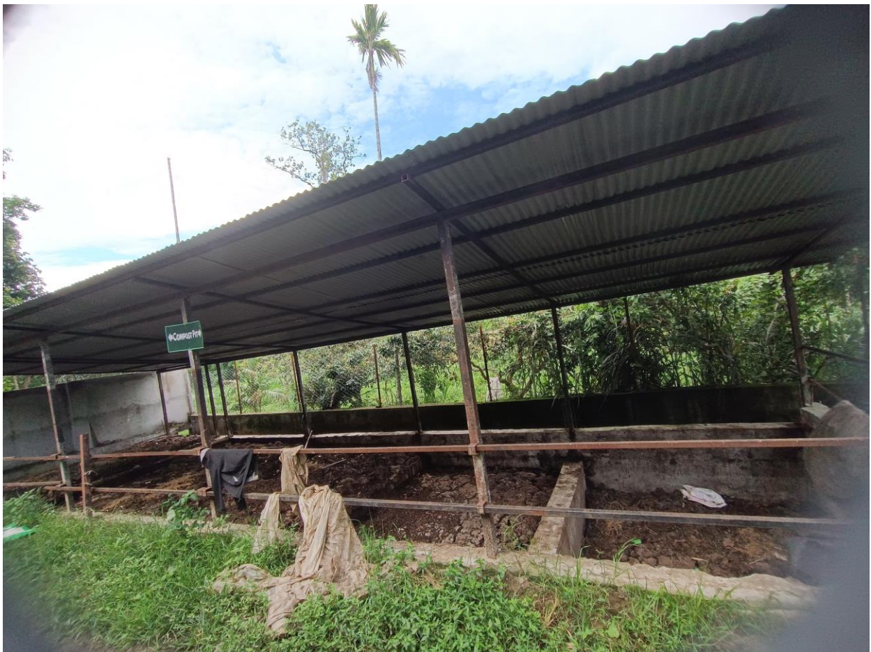
Shubhaagan Krishi Sahakari Sanstha Limited, Damak, Jhapa, Compost Pit
