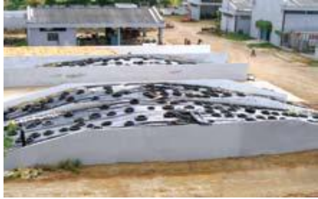
Figure 32: Covered surface silo
