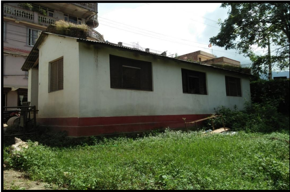
Existing Office Building to be Demolished
