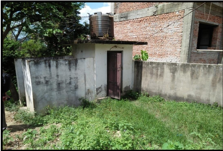
Existing Toilet to be Demolished
